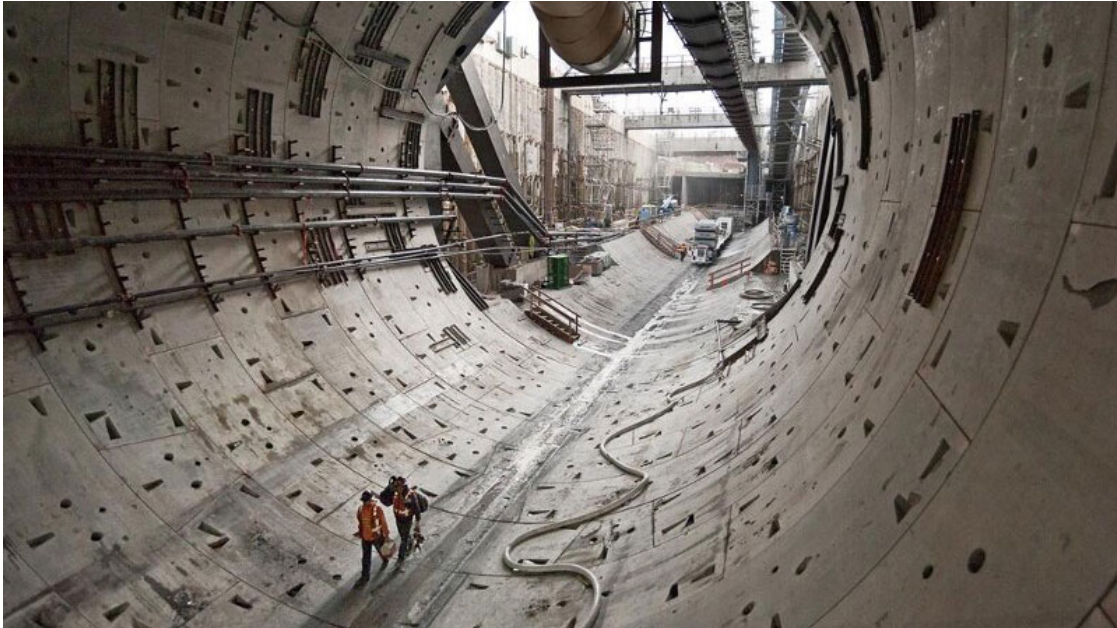
Just inside the expensively delayed Alaskan Way Viaduct Tunnel | Photo: WSDOT
