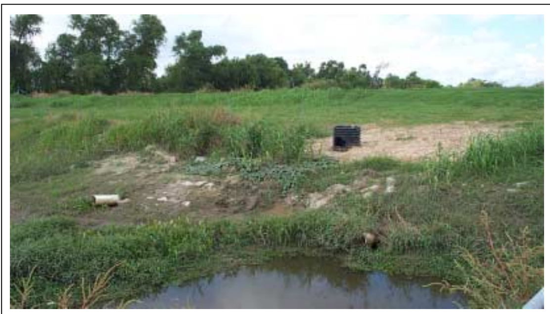
Fig. 2.2 A relief well was installed into the sinkhole at LSU Dairy Farm (August 2002).
