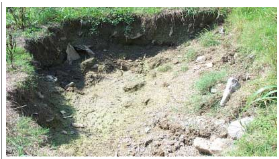
Fig. 2.1 A sand boil turned into a sinkhole at LSU Dairy Farm (July 2002). The sinkhole had been filled before, but reformed after several years.
