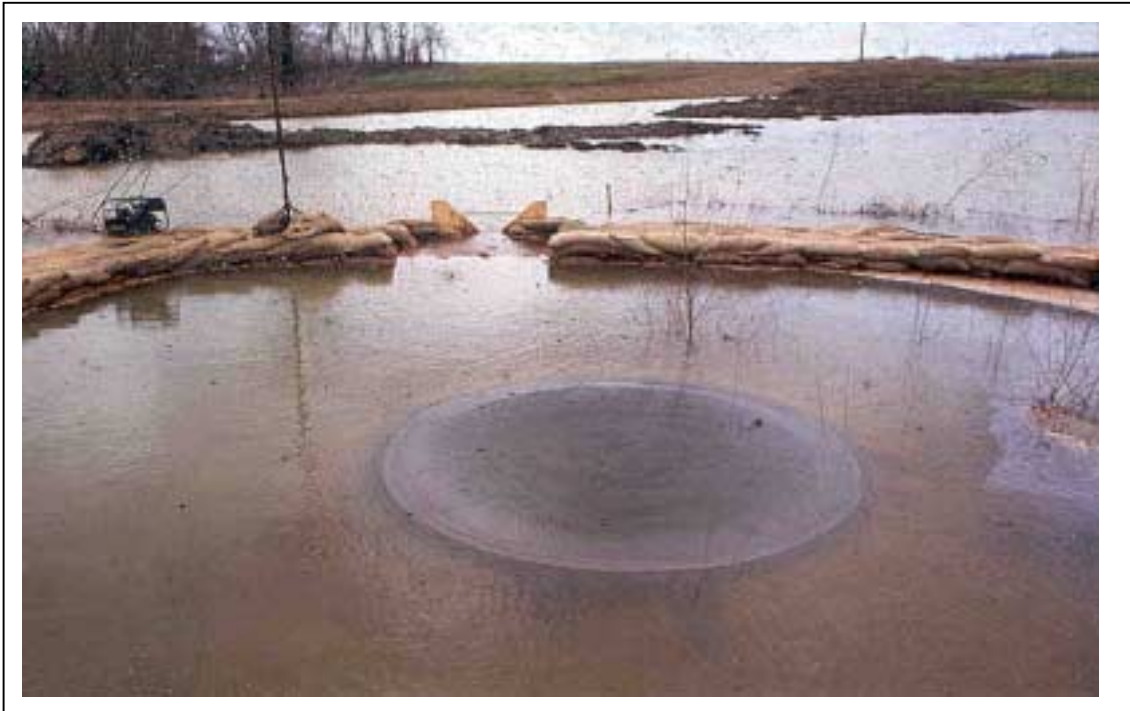
Fig. 1.2 A picture of a sand boil (source: USACE, Vicksburg District).
