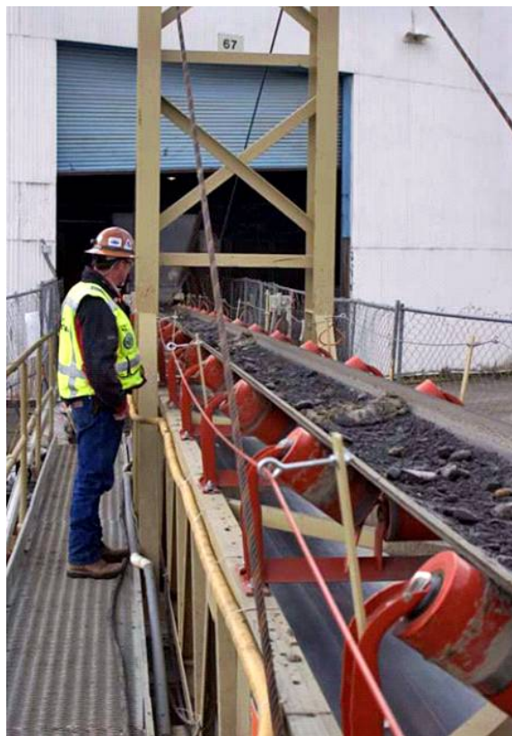
Figure 3-11 Typical Conveyor Transport of Excavated Soils
