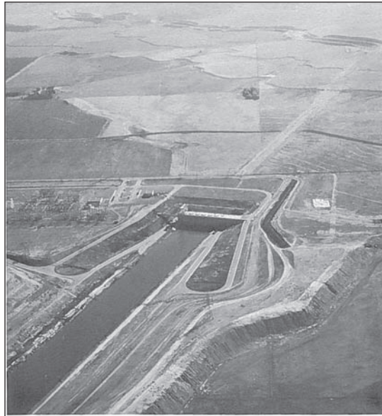
Tracy Pumping Plant
